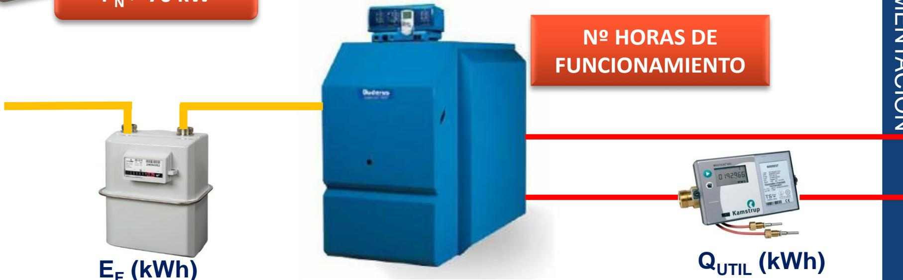
$$\eta_M = \frac{Q_{UTIL} \text{ (kWh)}}{E_F \text{ (kWh)}}$$
